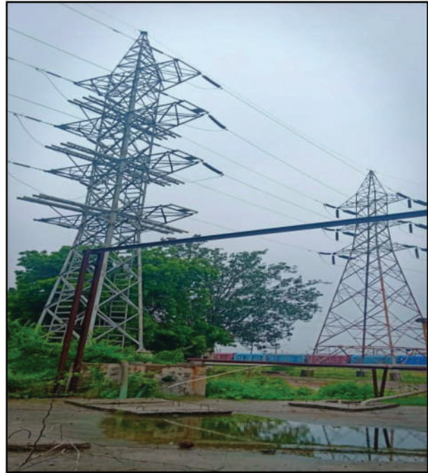
Tower erection and Stringing work by Torrent Power Limited at Vatva, Ahmedabad, Gujarat
